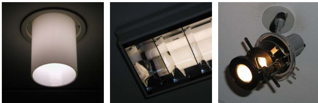
Figure 2.4: Common elements to modify the radiation pattern of a luminaire. Left: A lamp screen with diffuse transmission. Middle: Office lamp with reflective components. Right: Spotlight with polygonal aperture and projective lens.
